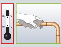
Clean all dust, dirt, oil and water from pipework using Armaflex cleaner where necessary. Install Armaflex Ultima self-adhesive when ambient temperature is between  $\pm 10$  and  $\pm 35$  °C.
